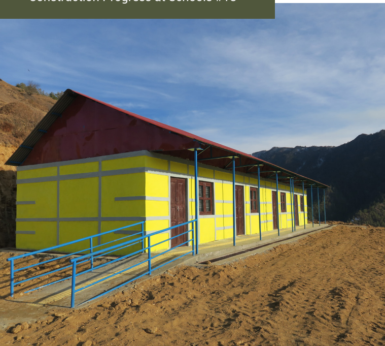
Construction Progress at Schools #18
