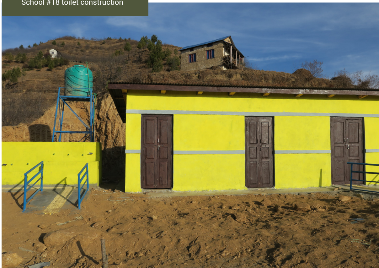
School #18 toilet construction
